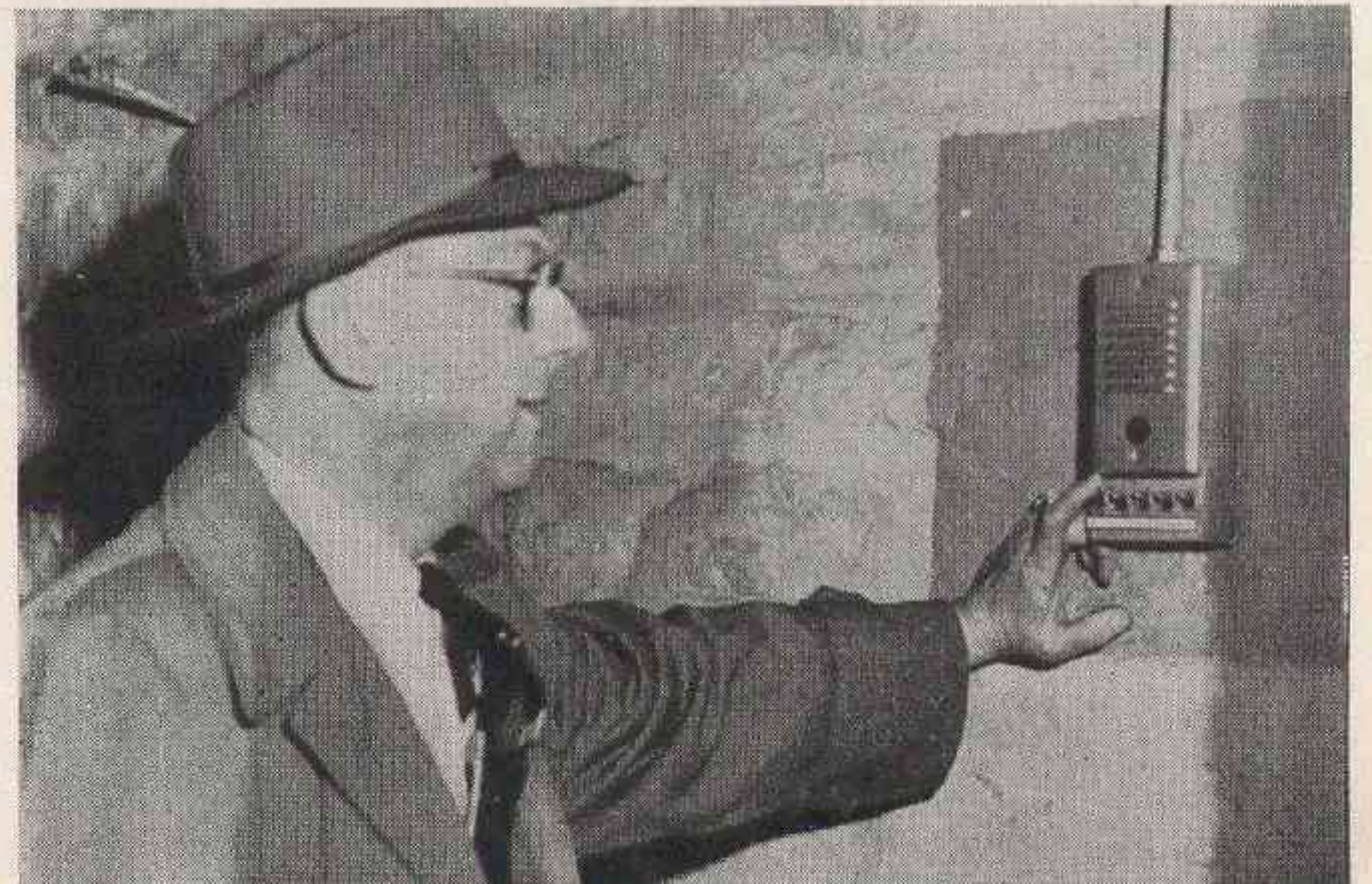
A FIVE-MASTER-STATION INTERCOM system, by Webster, is a time and step saver. A separate intercom setup, using two Webster Teletalks, connects the second-floor markers with first-floor loaders at the conveyor table.
