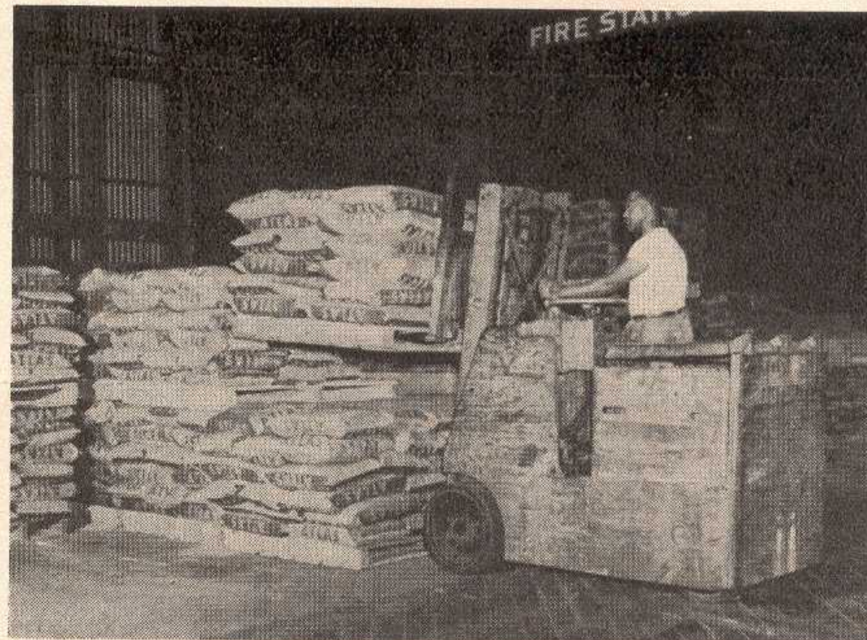
Some carload freight is handled at Pier 68, such as this palletized cement being stacked by an electric fork truck
