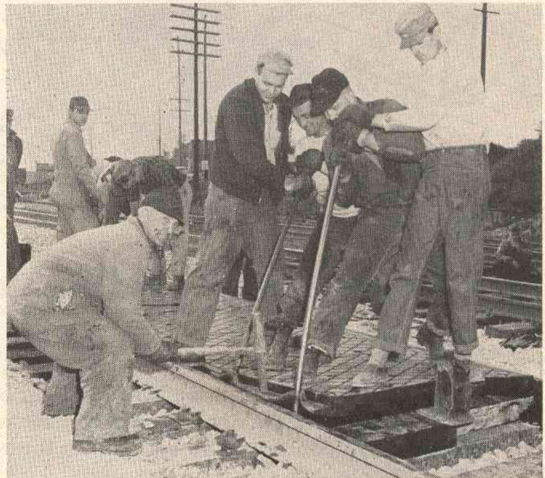
. . . FLANGE at the other end is sprung into place against web of rail to form a water-tight fit.
