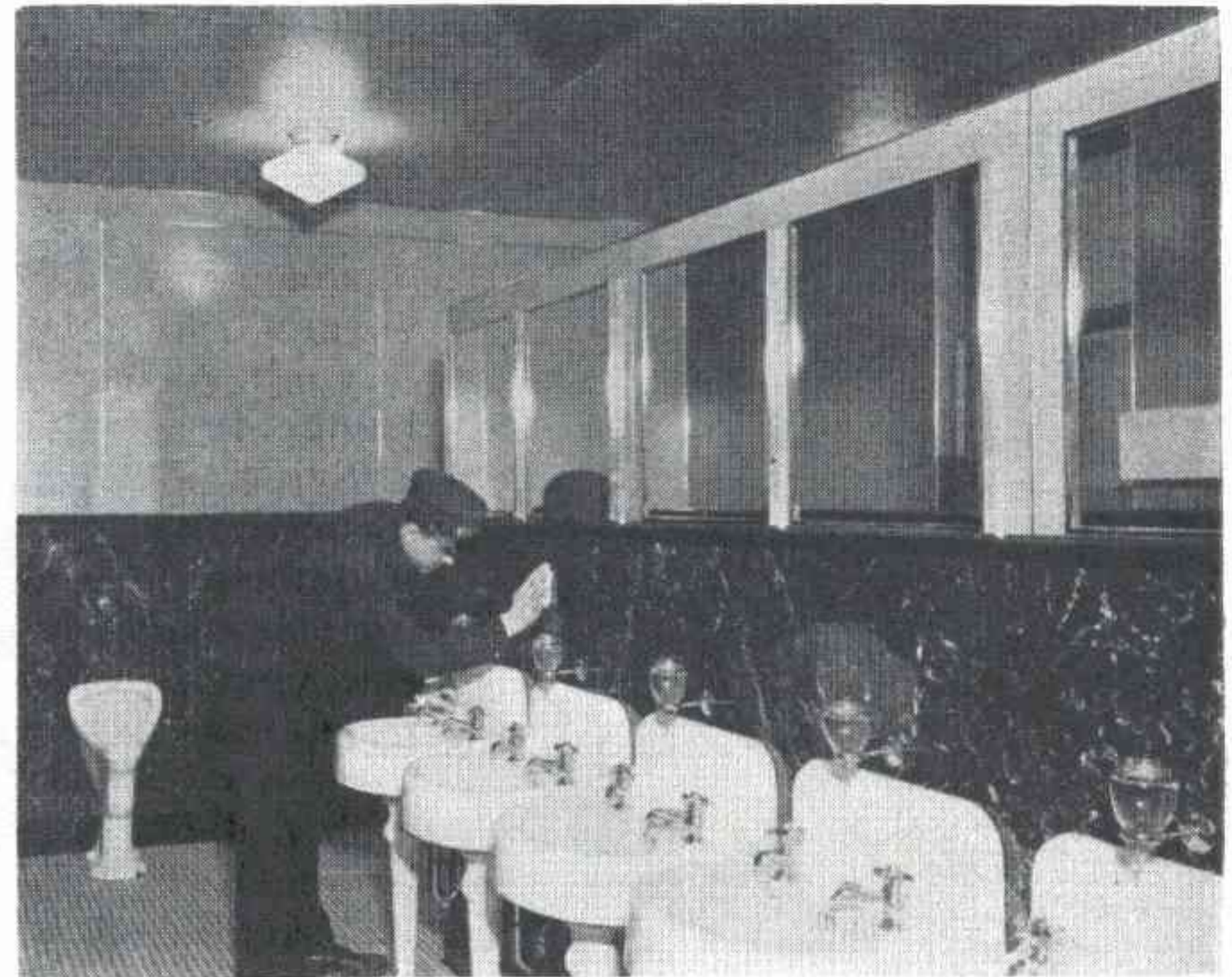
This View of a Portion of the Men's Room Is Illustrative of the General Character of the Improved Facilities
