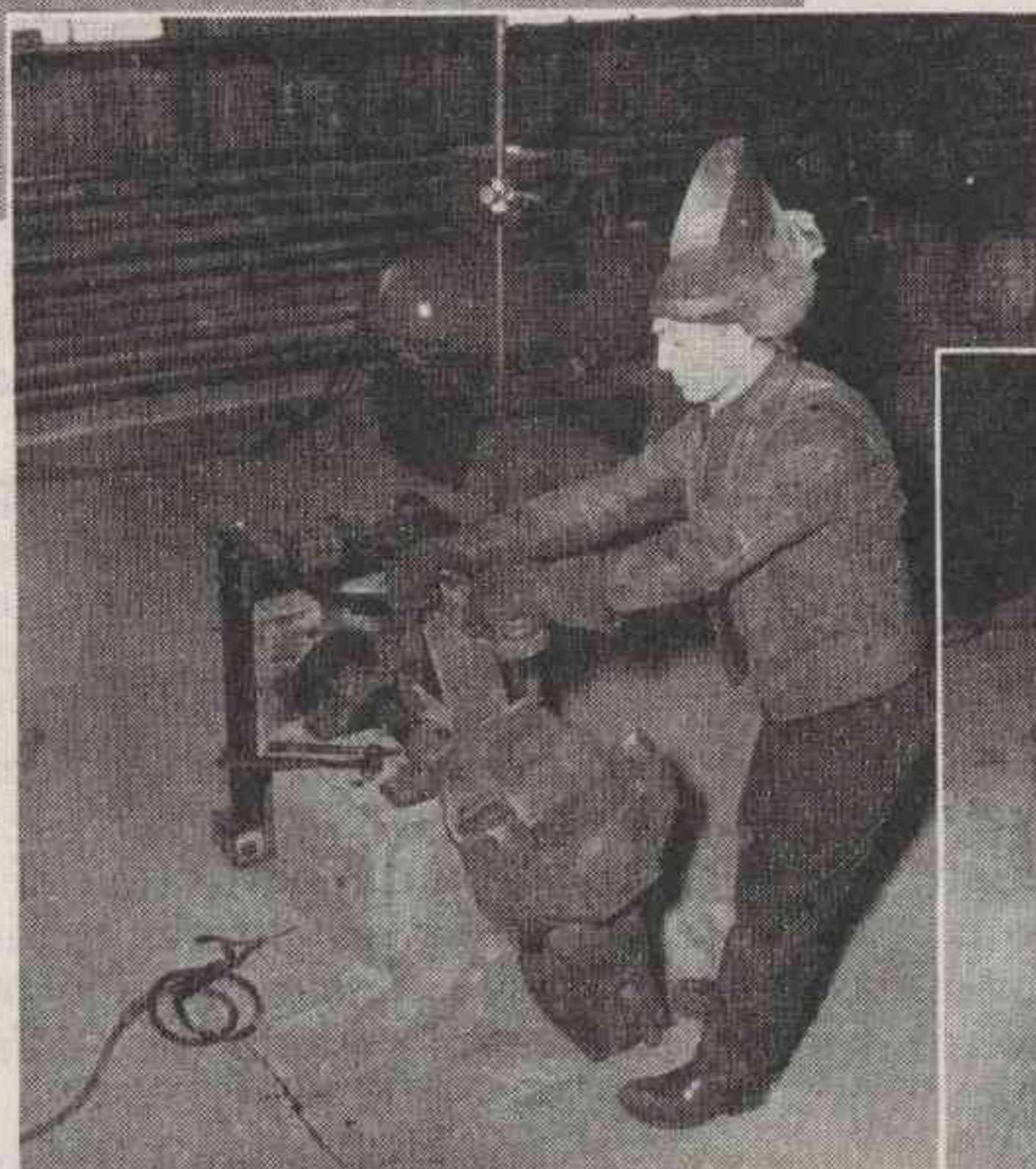
Three Steps in Welding Car Couplers—
