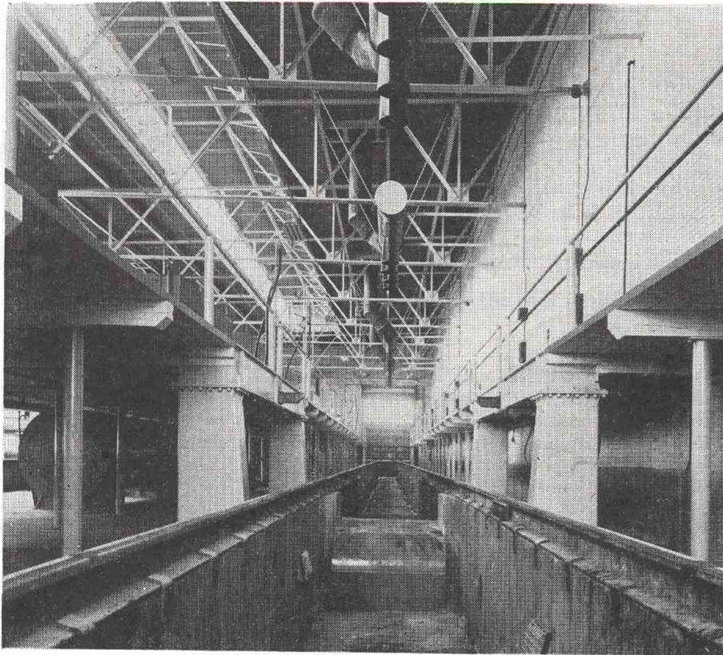
One of the pits in the service shop, showing body supports at drop table in "out" position—also overhead engine exhaust system
