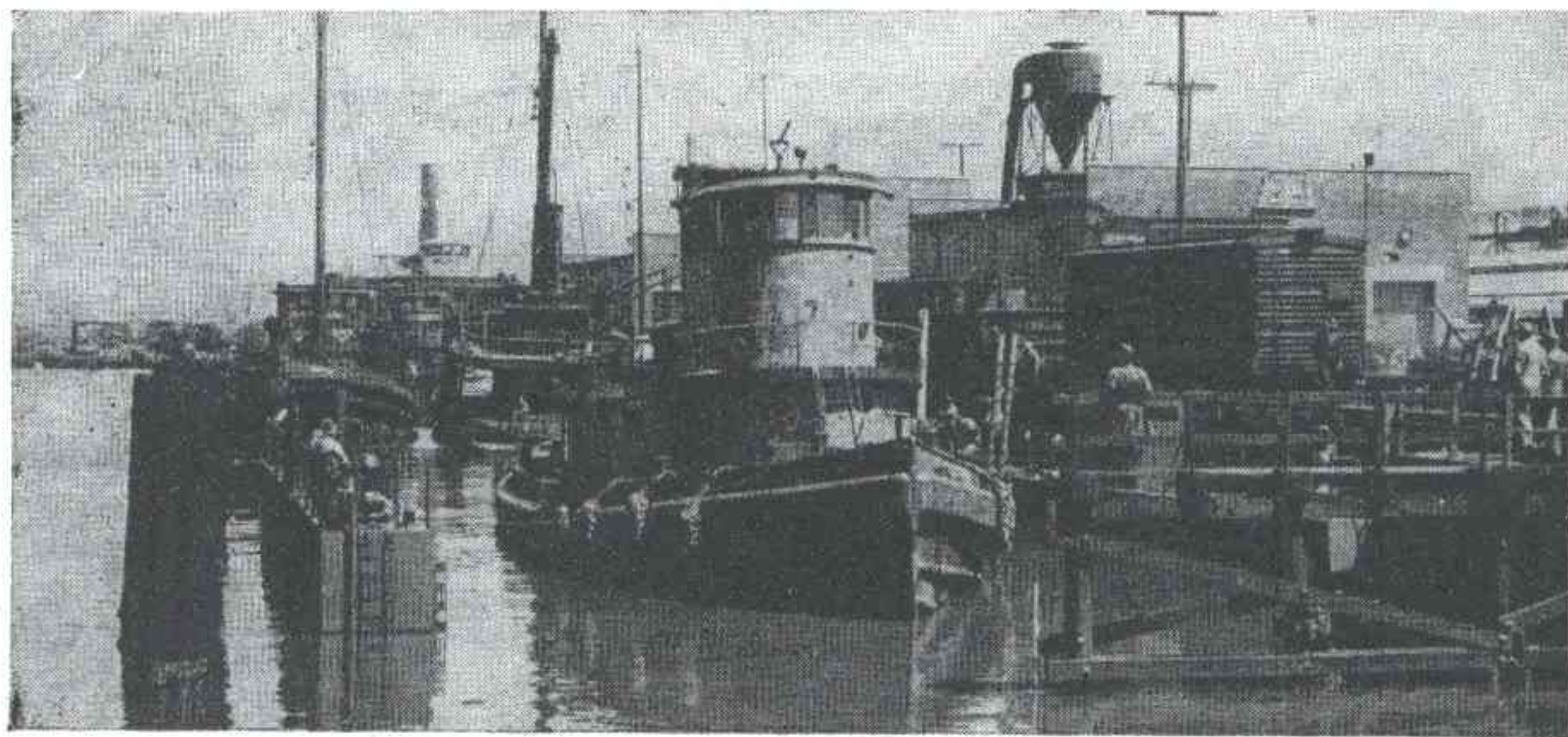
Left—A tug is maneuvered into position on the submerged dry dock for lifting
