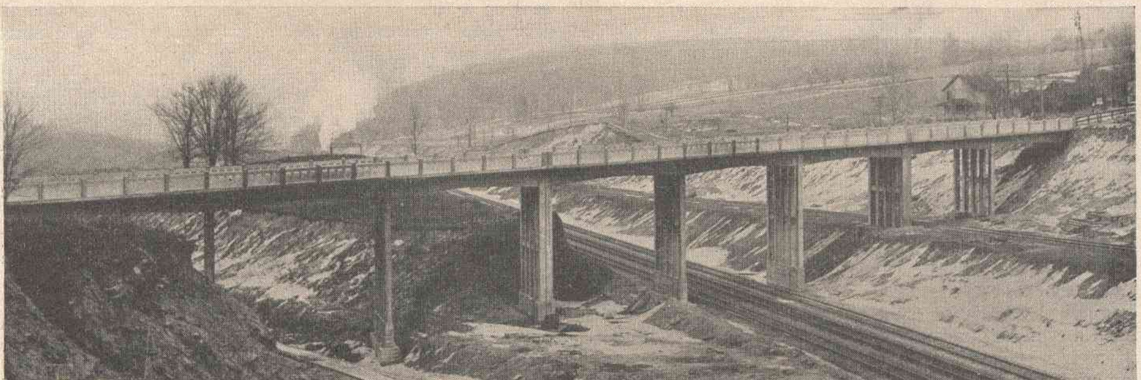
The Completed Viaduct
