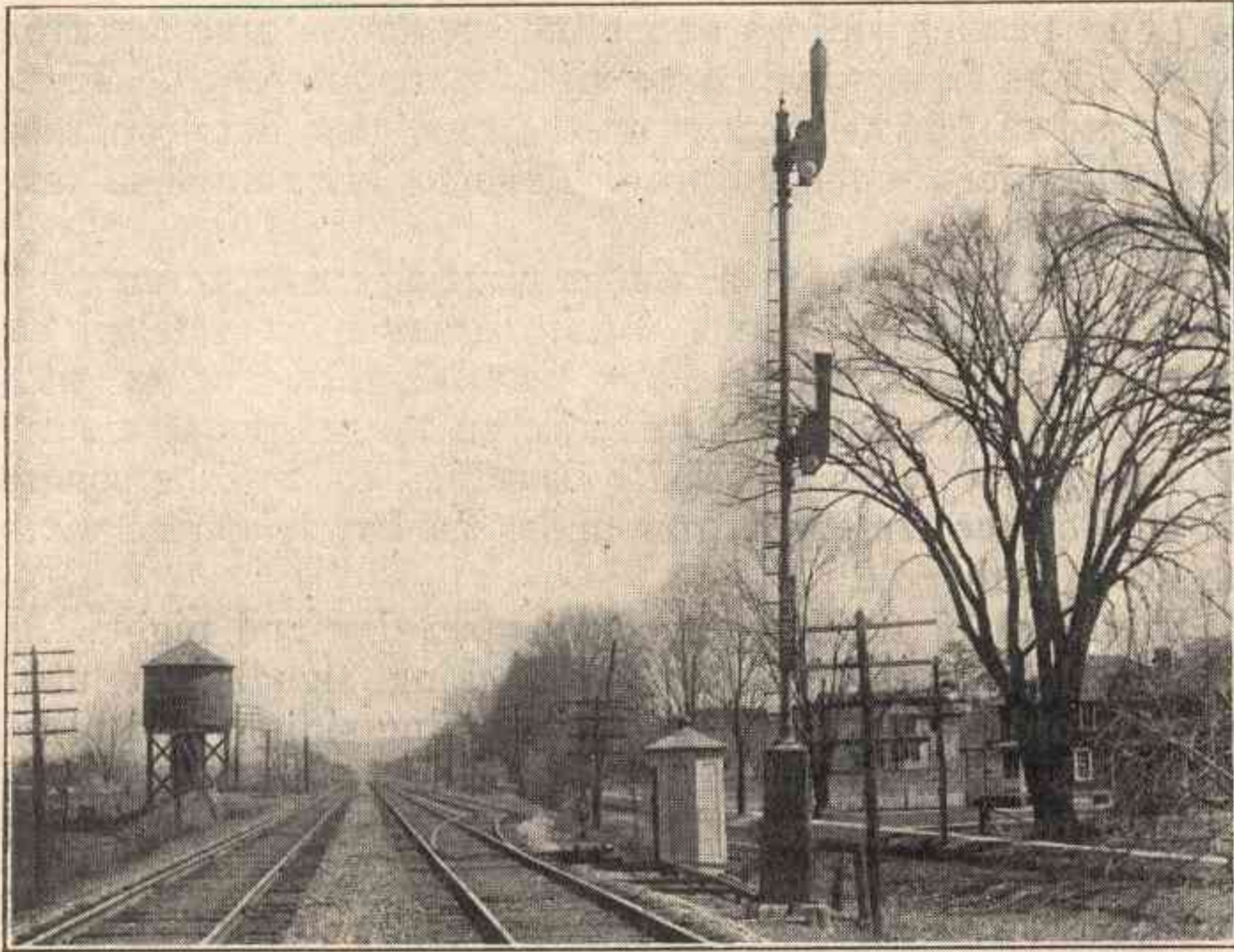
Automatic Block and Train Order Signal at Passing Siding L R
