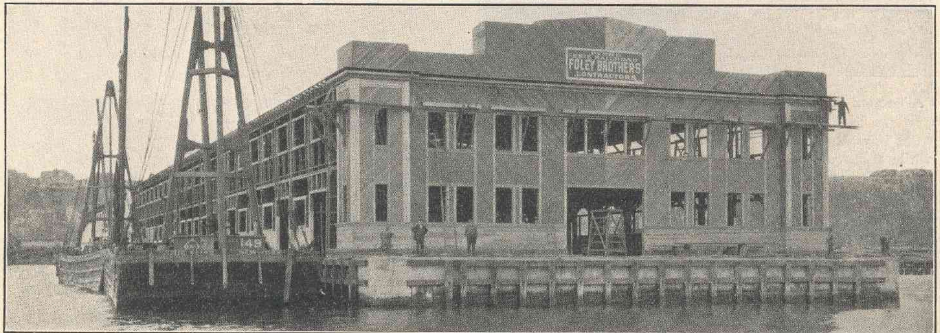
The Sheathing of the Pier Preparatory to Application of Zinc
