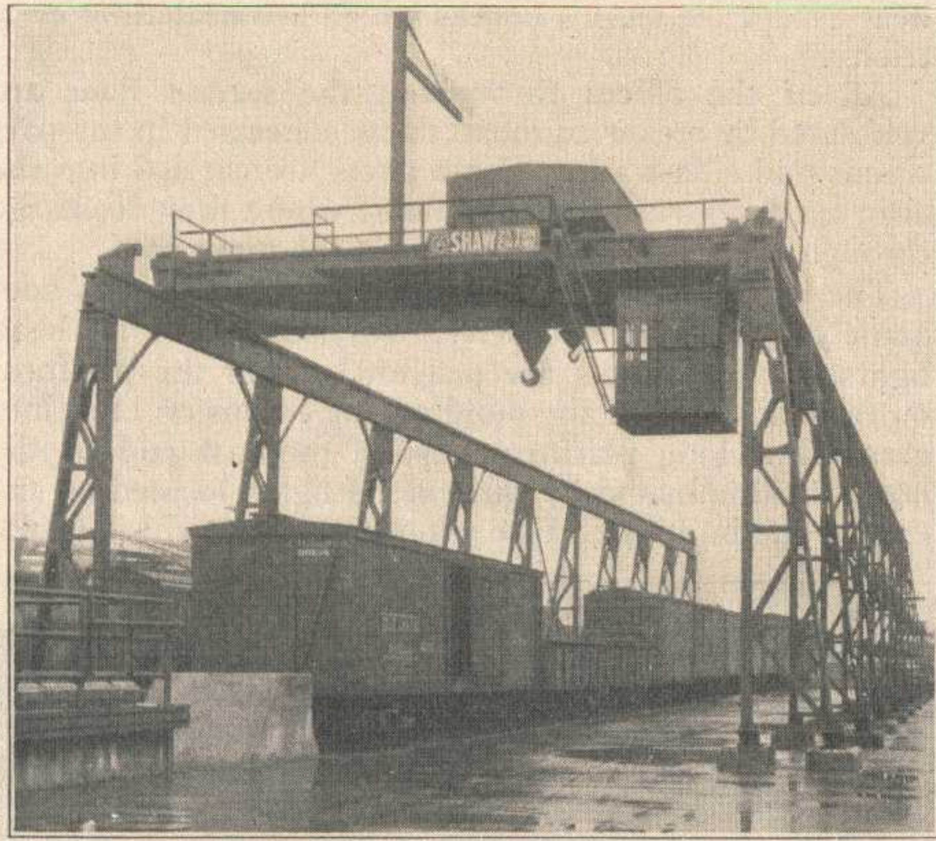
The 25-Ton Crane Which Serves One of the Team Tracks
