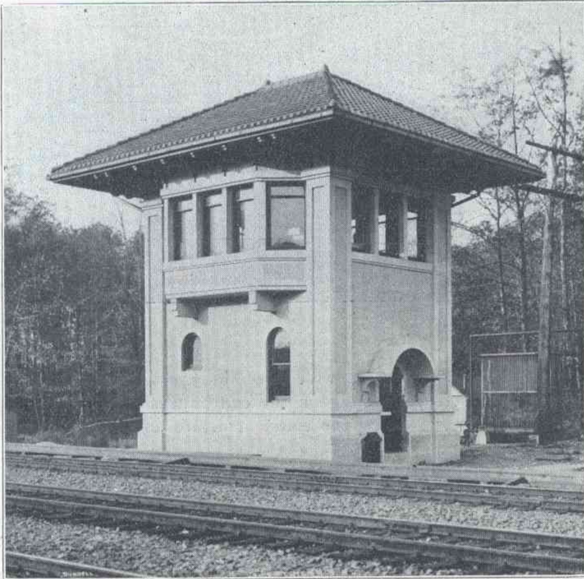
Standard Concrete Signal Tower at Port Morris, N. J.
