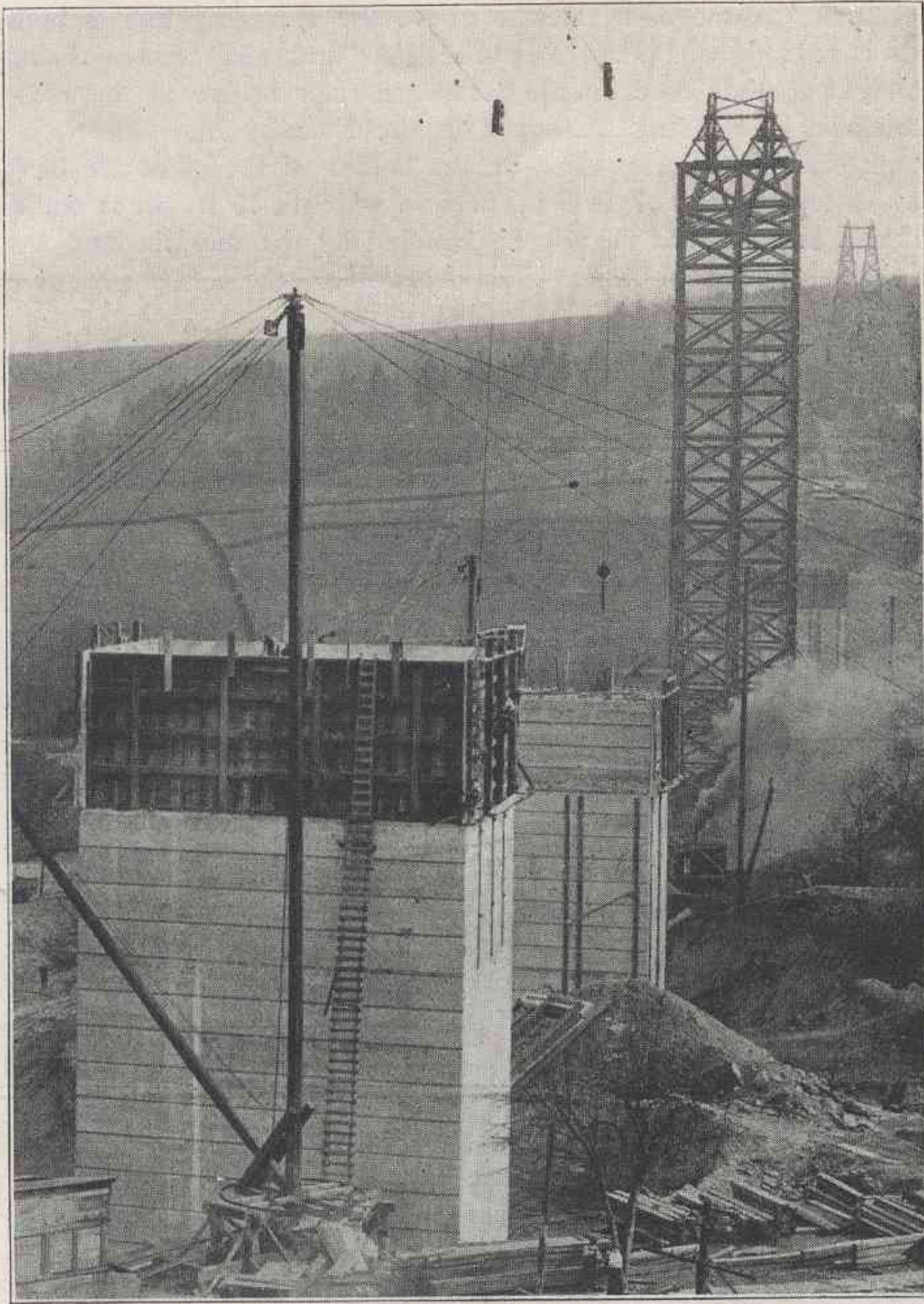
Showing Sectional Pier Forms and Double Cableway.
