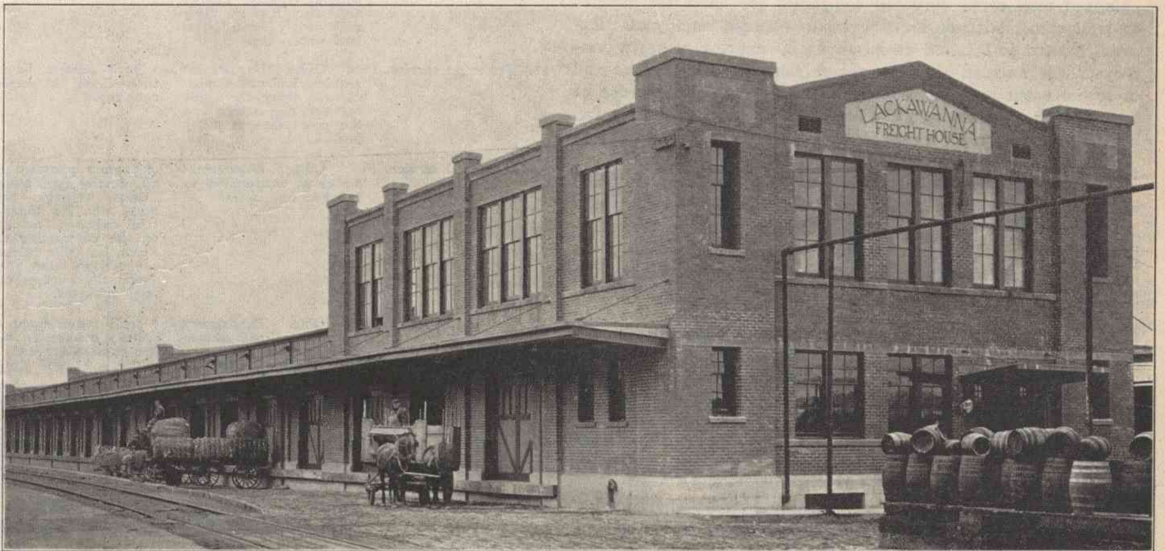
New Inbound Freight Station on the Lackawanna at Utica, N. Y.
