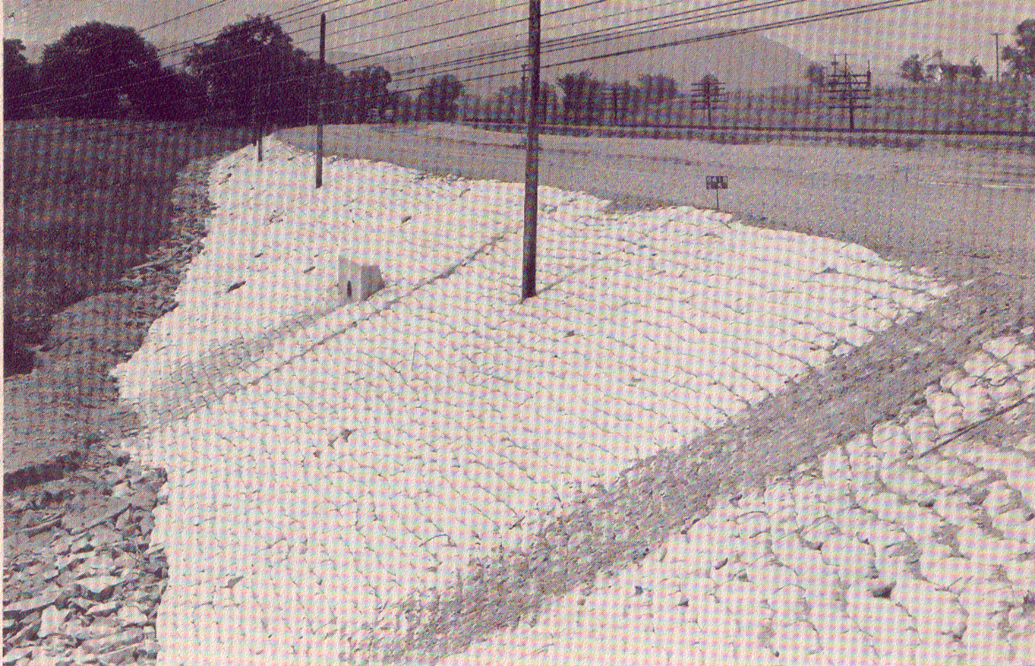
BAGGED CONCRETE, pinch batting for unavailable stone on Erie relocation project . . .
