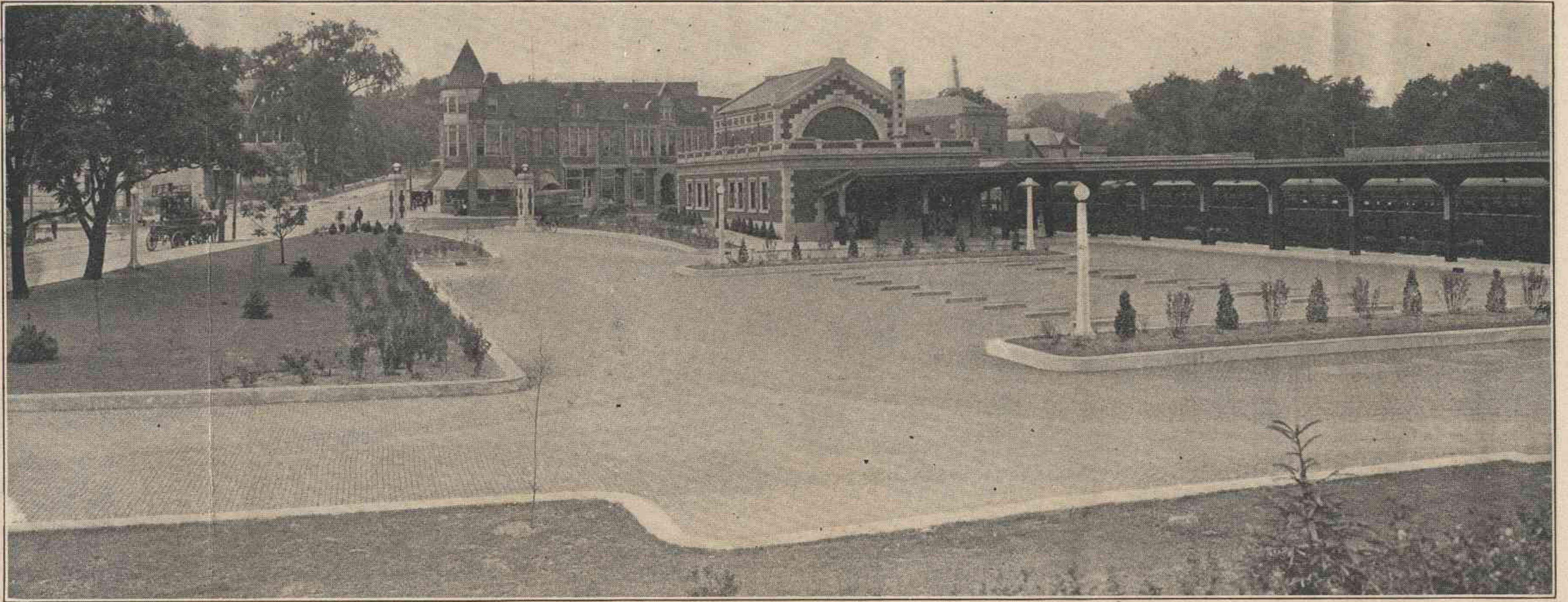
Fig. 3—Rear View of Montclair Station and Driveways.
