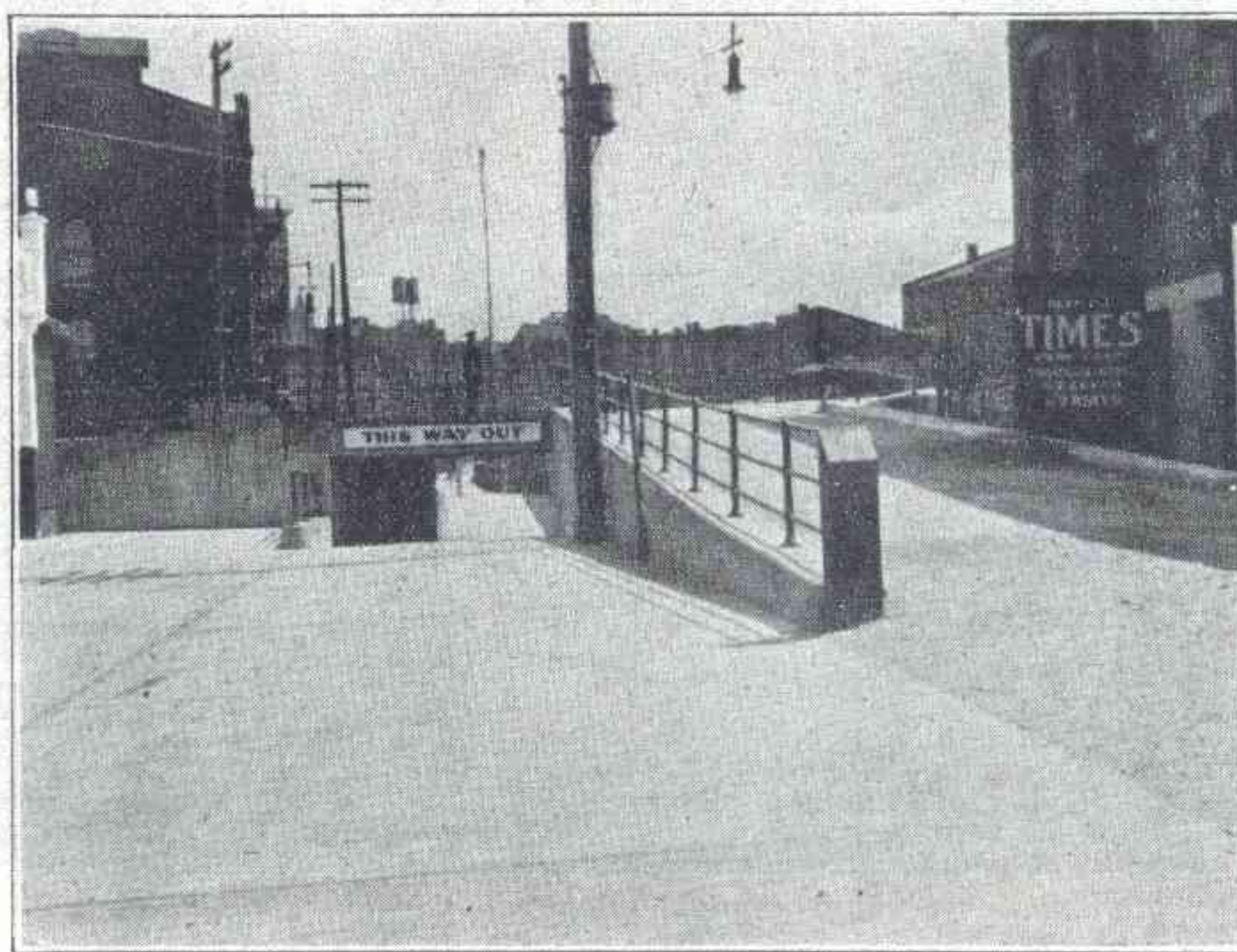
Looking North from River. Concrete Pavement in Front of Dock House in Foreground.
