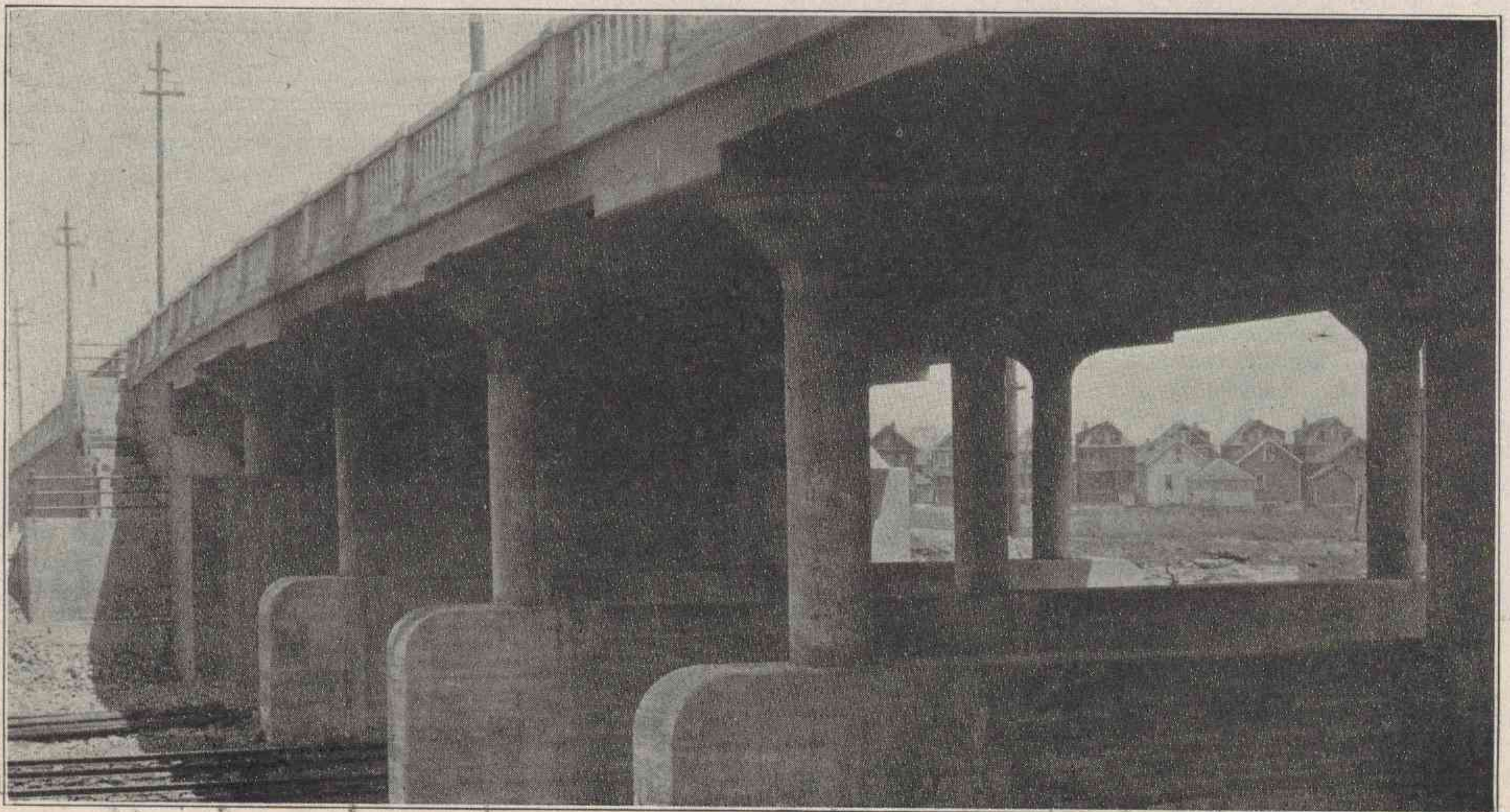
Kensington Avenue Viaduct Showing Columns and Collision Base for Bents.
