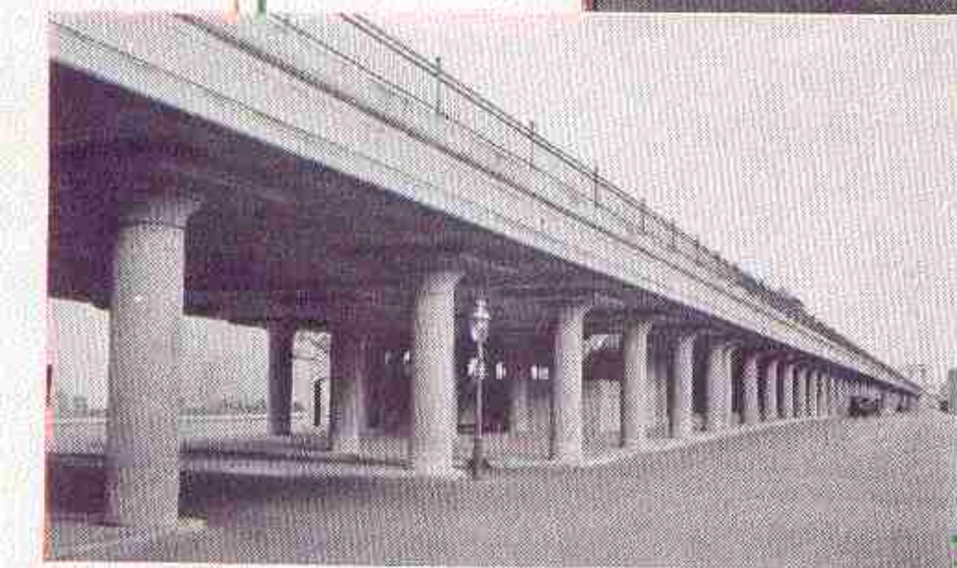
A viaduct in the Oranges—a remarkable engineering accomplishment.
